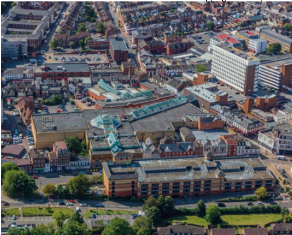
Figure 2 (below) is another aerial view from the north. The Car Park site is in the foreground, with the glazed roofs of the malls for The Galleries and the Arcade Shopping Malls beyond.
